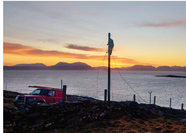
Power being restored after storm Eowyn
